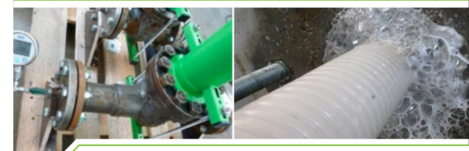
Leak test under real gas and on a wall duct (l.t.r.)
